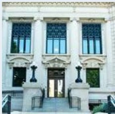
Historic Illinois Supreme Court Building reopens after 13-month restoration
